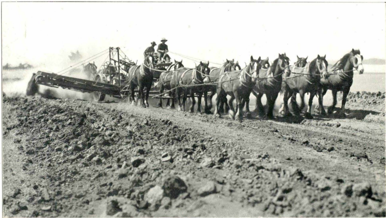
EXCAVATING IRRIGATION CANAL.
