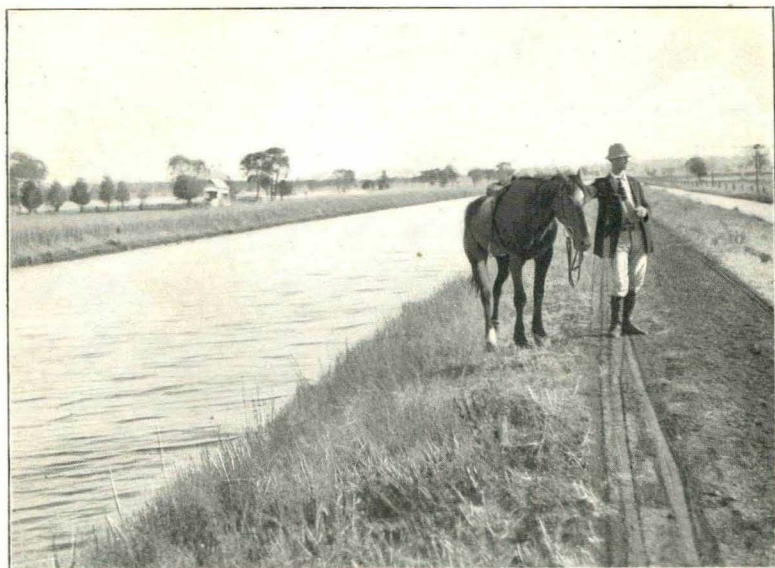
A MAIN IRRIGATION CANAL.
